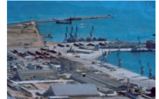
Castellón - WSF, logistics (Spain)
